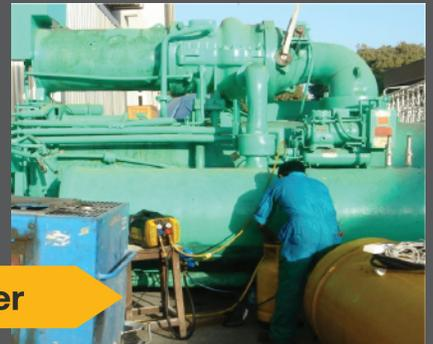
Chillers containing 4000 lbs of R-134A being recovered with a G5Twin in the intense heat of Saudi Arabia. What once took a week, now only takes only 18 hours with the speed and reliability of the G5Twin.
